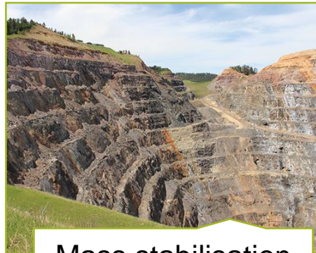
Mass stabilisation and erosion control
